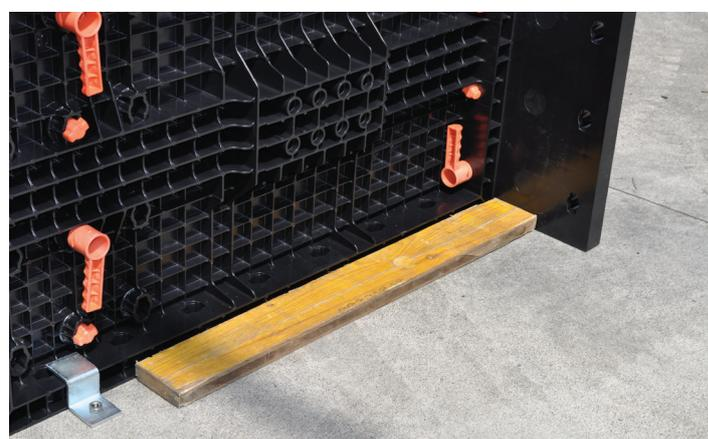
The anchoring to the ground is useful to avoid lifting of the formwork and it is done using metal or timber brackets.
